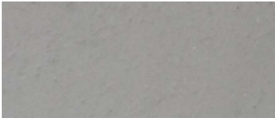
Wall with RenderCon 5S after 10-days (picture taken closely to show the finish)
