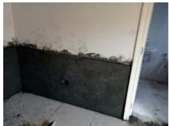
Plaster applied and ready for taking halogen light (after setting).
