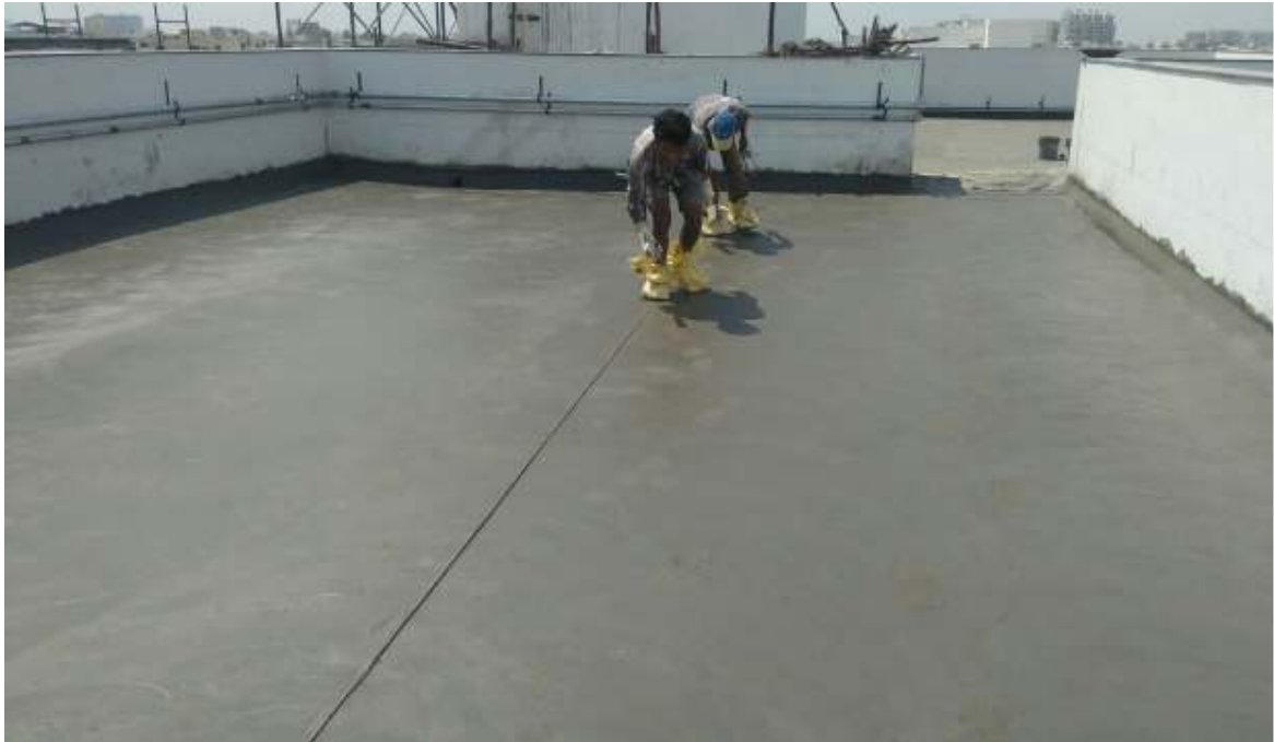
Cutting grooves for grid lines
