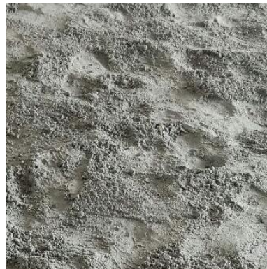
Dry Mixed (Cement + Sand)
