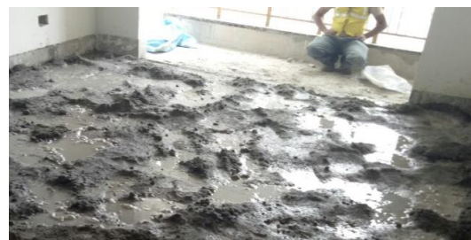
Mixing More Water, Ensuring no cement / Sand particle is dry.
