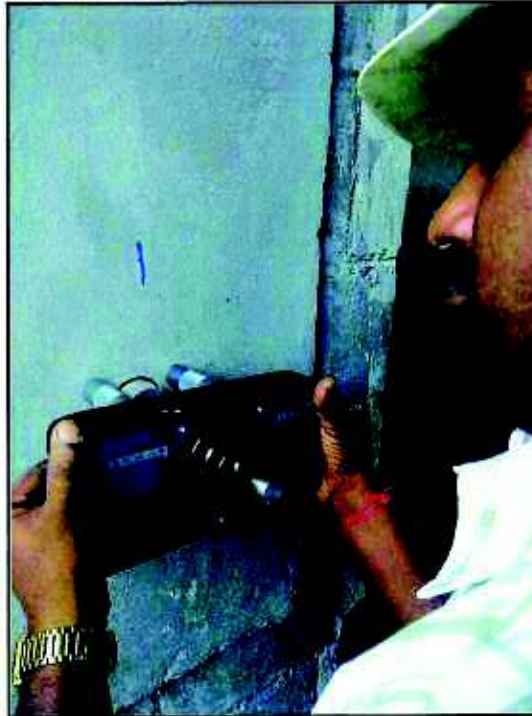
View of Pull-off test
