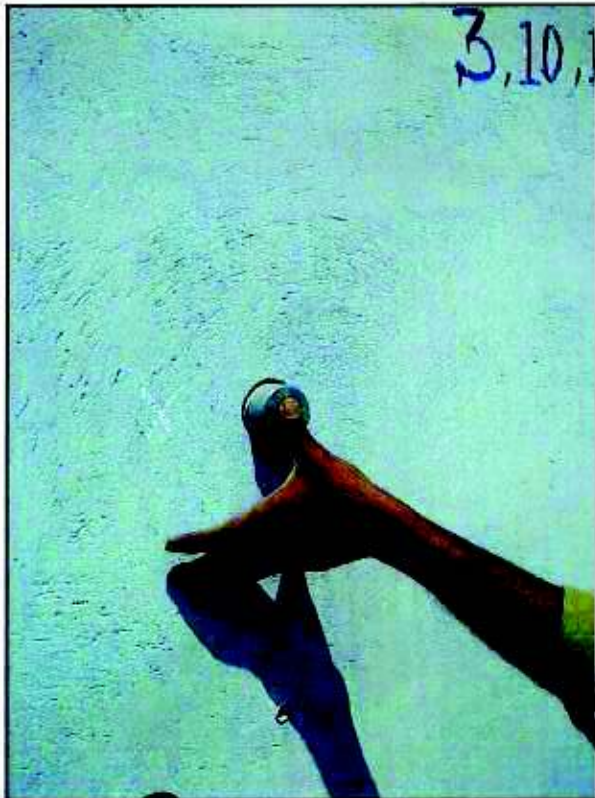
Fixing of test discs in progress
