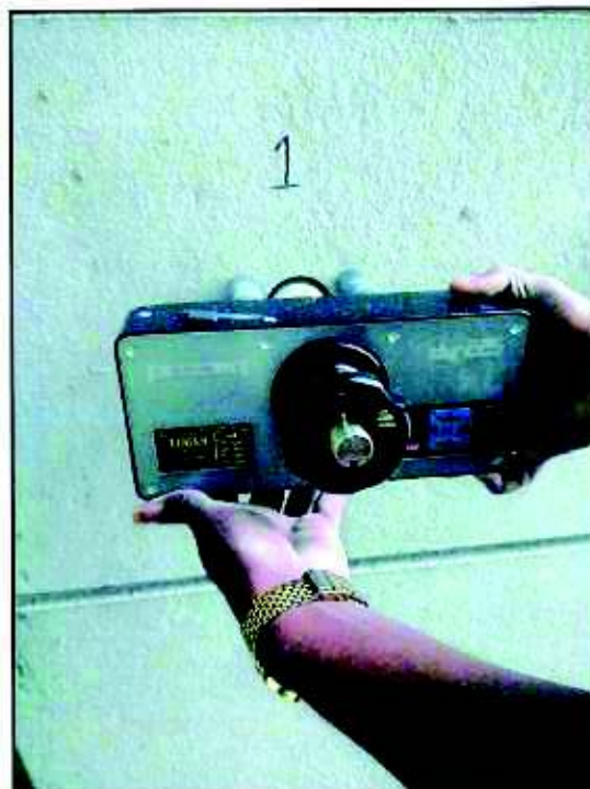
View of pull-off test
