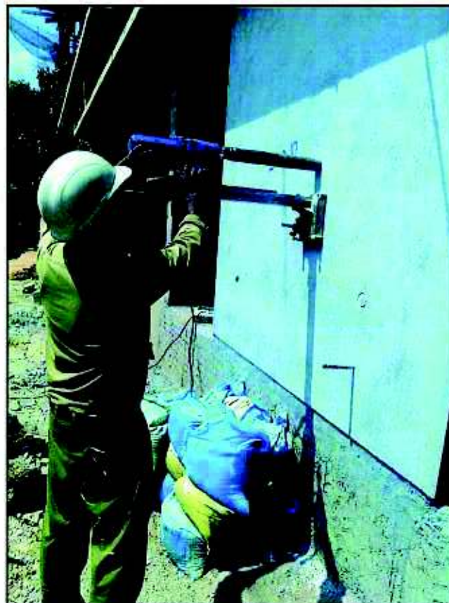
Making of groove in progress
